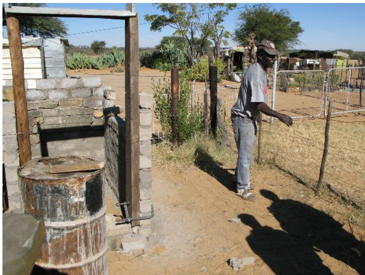
Photo 14: Joseph Ganeb building a latrine
